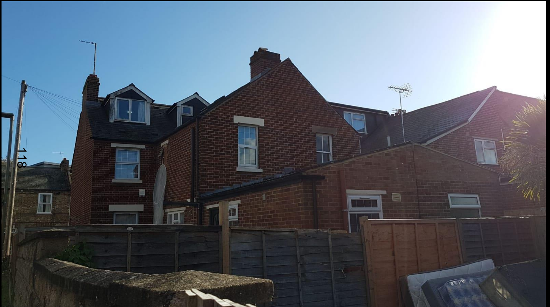
Rear of properties on East Avenue
